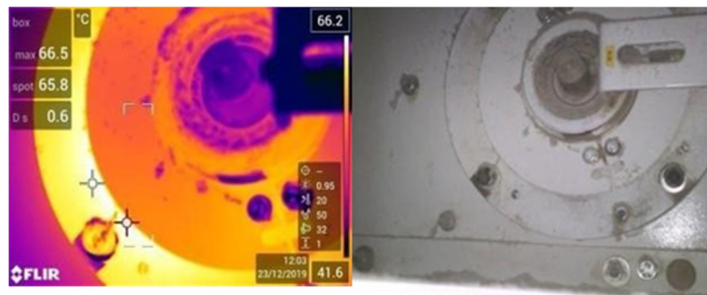
Figure 5. opening roller bearing housing at card no-3 a) IR Image b) Visible Image
