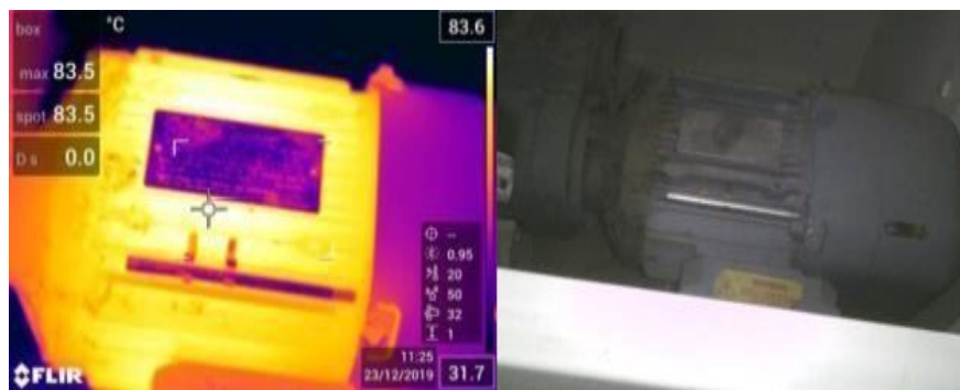
Figure 1. Belt motor found a heated condition at bale Plucker a) IR Image b) Visible Image
