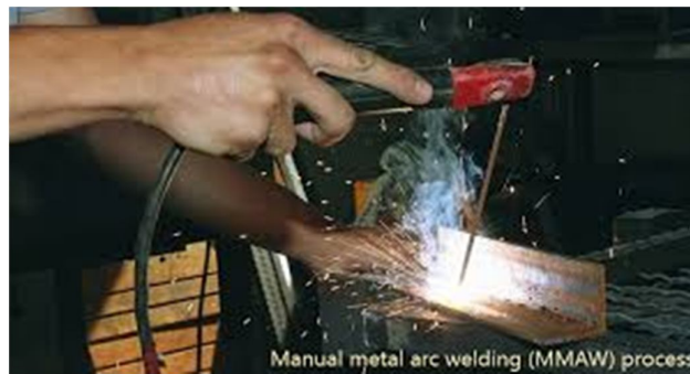
Fig 5. Welding the angles together
