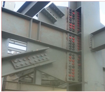
Figure 8a. Special concentric brace frame connection detailing
