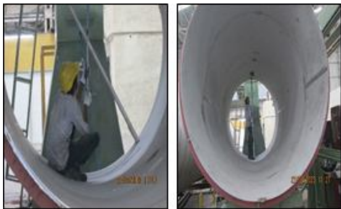
Figure 3. Purging Operation
