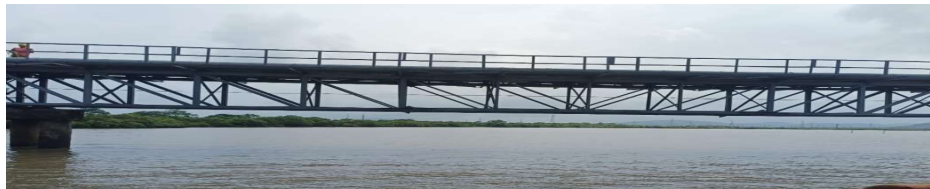
Figure 1 N-Type Steel Footbridge
