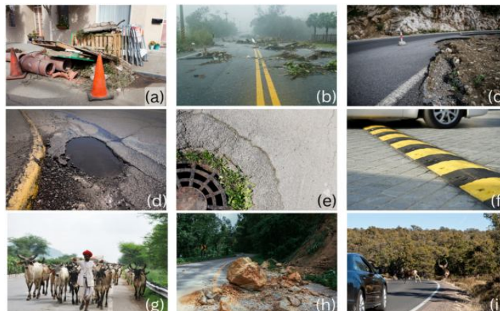
Figure 2: (a) Road Maintenance Objects & Construction Debris, (B) Debris Fallen on The Road, (C) Road Surface Failure, (D) Potholes, (E) Maintenance Holes, (F) Speed Bump, (G) Farm Animals on Road, (H) Landslide Debris, (I) Wild Animals Crossing the Road
