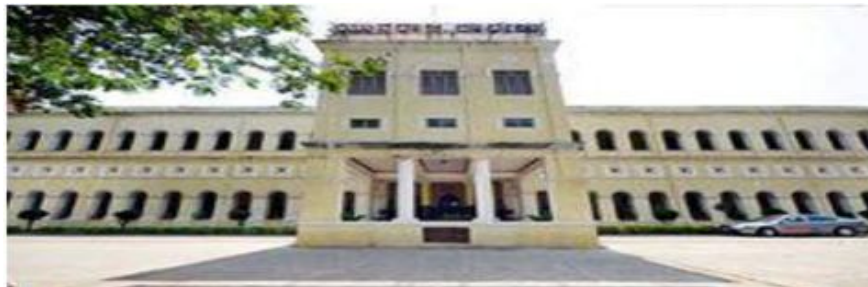
Figure: 5 Front view of Yuvaraja College of Mysore for which Seismic evaluation is performed
