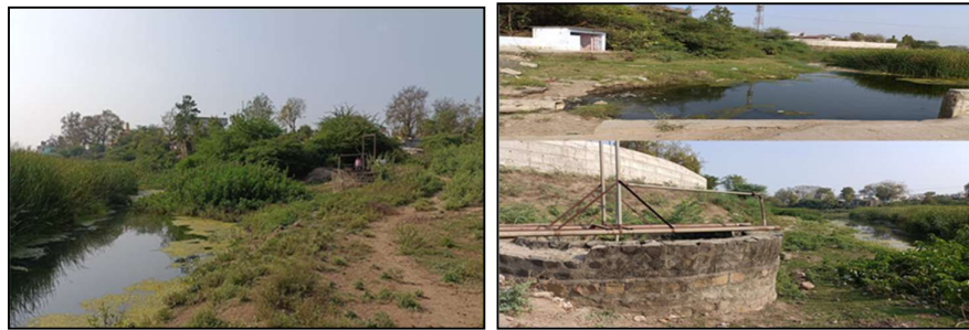
Figure 3 Existing sewer condition of Dhapewada (Source: site visit image captured by author)
