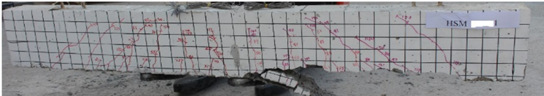
Figure 1- Beam REMB before Rehabilitation
