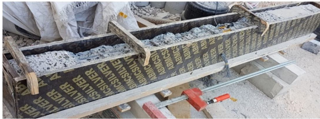
Figure 2-Form work for concreting
