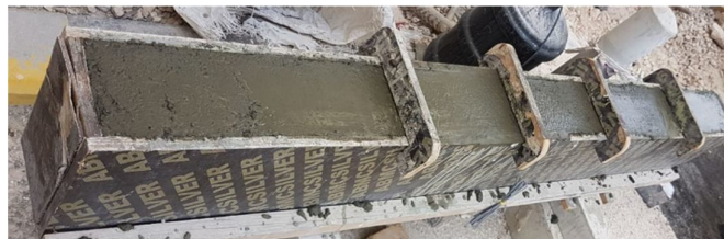
Figure 4-Post compaction of concrete
