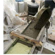
Figure 5-Bonding Agent and Micro-concrete
