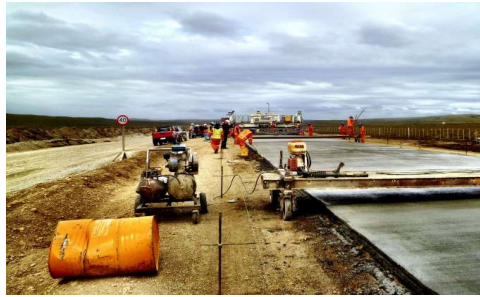
Figure 4. Construction work going on with FRC at Sombrero Highway, Chile
