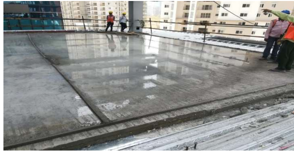
Figure 6. Metal/Composite Deck application at a project site in Hyderabad, India
