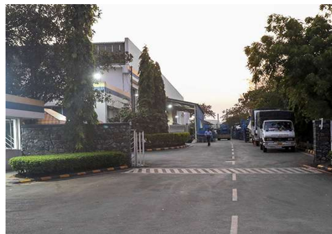
Figure 5. Internal Road works for Factory in MIDC Pune
