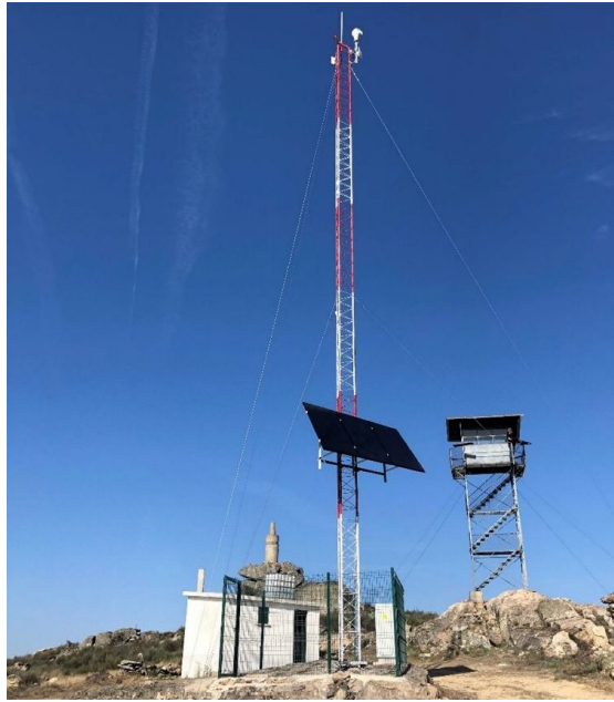
Figure 2. Remote data acquisition tower (autonomous energy and communications)
