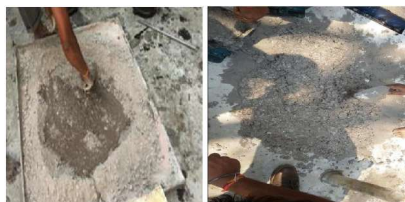
Figure 3. Mixing of Geopolymer concrete
