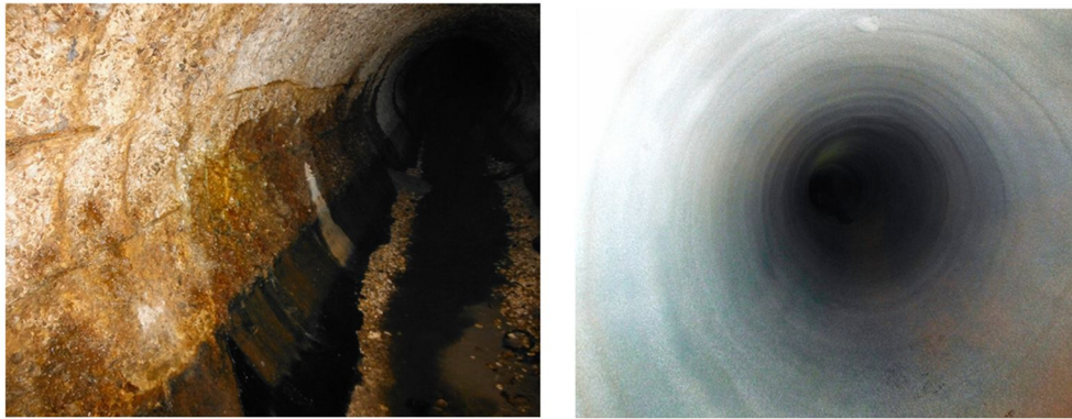
Figure 7. A study of the sewer pipe condition: prior to and following rehabilitation
